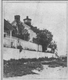
THE SOUTH CORNER The stone is within the sea wall.
